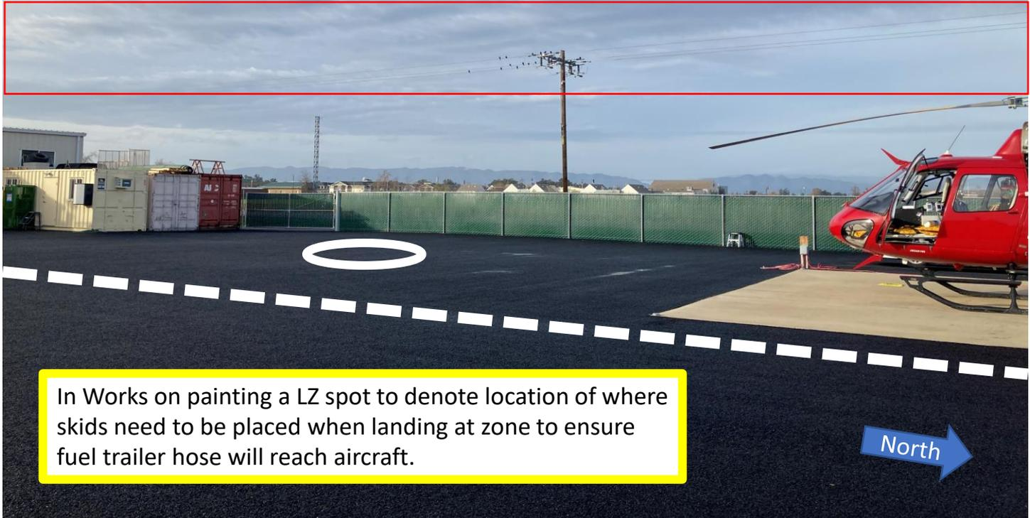
In Works on painting a LZ spot to denote location of where skids need to be placed when landing at zone to ensure fuel trailer hose will reach aircraft.
